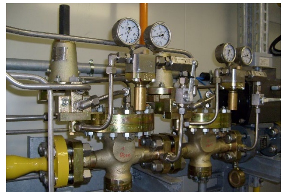
High Pressure Monitor Regulators for 150 bar on underground gas storage
