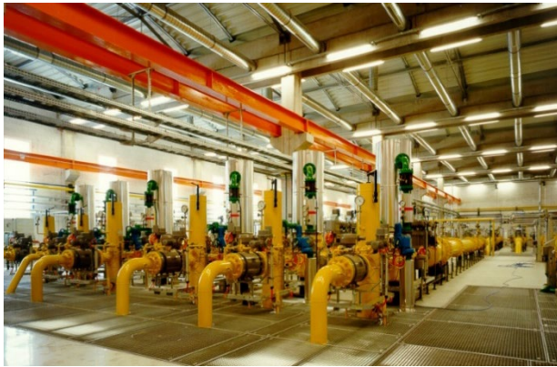
City gate station in a concrete building with hot water heating from hot water boiler system: Flow: 3 x 60.000 & 3 x 80.000 nm 3 /h Pin: 38 – 70 bar Pout: 3 – 4 bar
