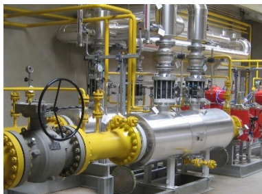
Gas Preheater WAT-LW Gas Flow 150.000 nm 3 /h; PN70
