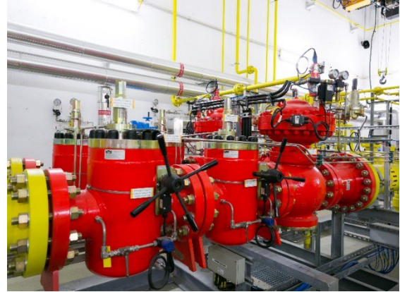
DN200 (10") PN100 – Double SSV + Regulator for power plant
