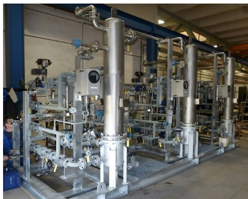
Aqueous ammonia vaporizer skids for coal power plant
