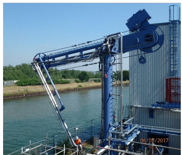
Aqueous ammonia ship unloading facility for a coal power plant
