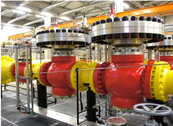
DN300 (12") PN100 – Monitor Regulation for main gate city station
