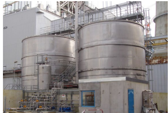
Aqueous ammonia storage tanks for coal power plant
