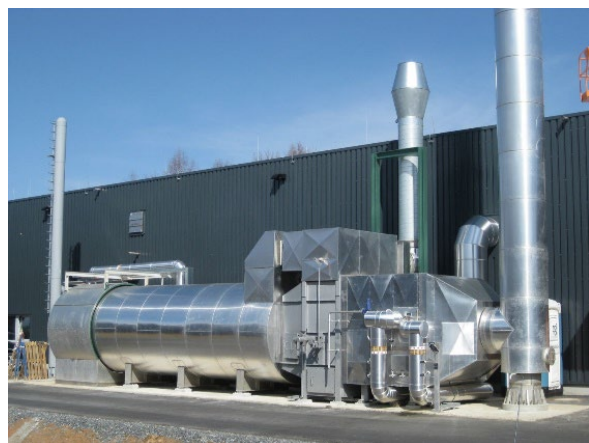
TNV for exhaust air from coating plant, 13.000 Nm 3 /h; Pollutants: Petrol, 5 – 160 kg/h
