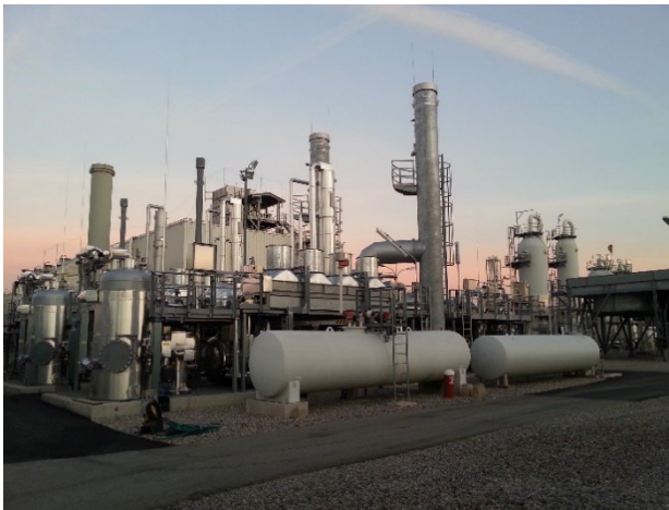
GDU on country border Compressor Station Gas flow: 9.600.000 nm 3 /d Pin: 35 – 70 bar TEG-flow: 6.500 kg/h
