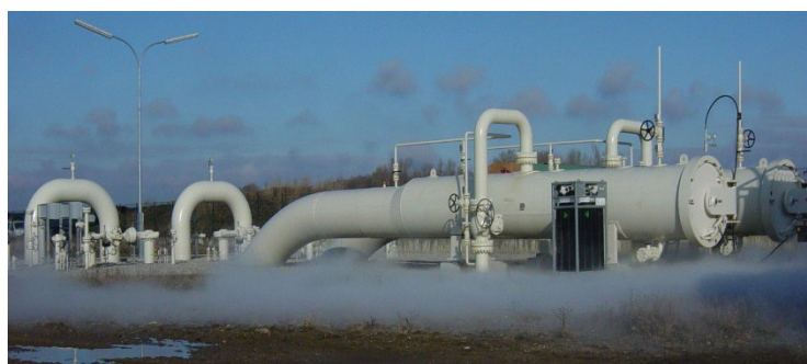
Pig Trap with HEAT Quick Opening Closure DN 1400/1600 (56"/64"); PN100
