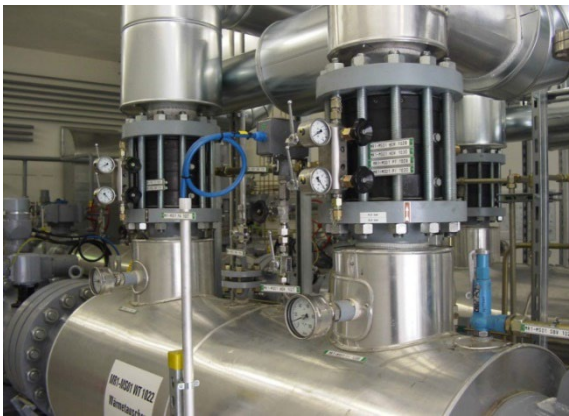
Warm Water Safety Shut Off Valves G42 – 1"-10"; PN40 – ANSI1500
