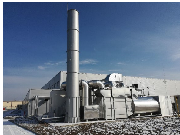
Concentrator with TNV for exhaust air from surface treatment processes, 70.000 Nm 3 /h; Pollutants: Xylol, Toluol; max. 1.100 mg/nm 3
