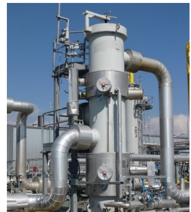
Filter Separator SNP Gas Flow 280.000 nm 3 /h; PN84
