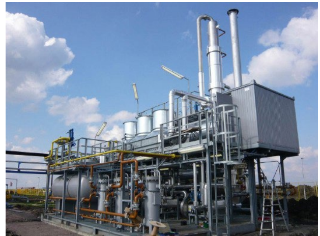
GDU on Underground Gas Storage Gas flow: 5.000.000 nm 3 /d Pin: 45 – 87 bar TEG-flow: 8.000 kg/h
