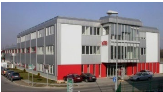
Office building and fabrication workshop
