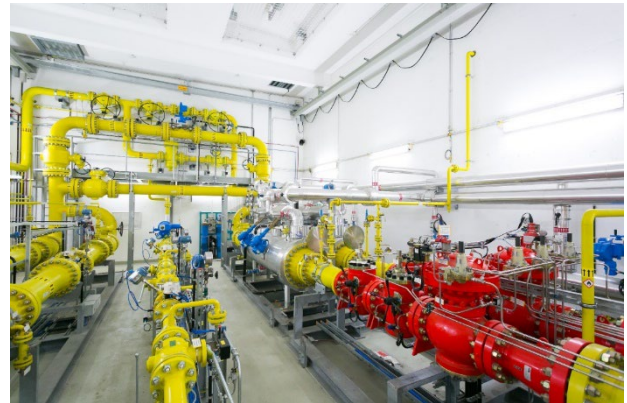
FGSS on skid with erection at site in a concrete building with hot water heating: Flow: 150.000 nm 3 /h Pin: 38 – 70 bar Pout: 31 – 33 bar & 3 – 4 bar
