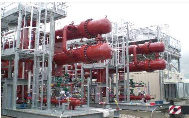
LTS unit gas production plant Gas flow: 2 x 1.000.000 nm 3 /d Pin: 45 – 80 bar
