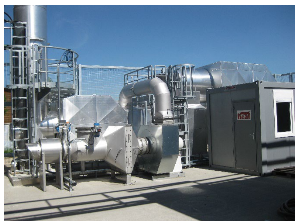
KNV for exhaust air from synthetic fibre production 13,000 Nm 3 / h; Pollutants: IPA Hexane; max. 52 kg/hr
