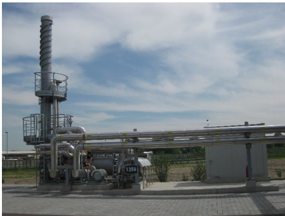
TNV for exhaust air from research facility, 400 m 3 /h Pollutants: various VOCs; 19 kg/h
