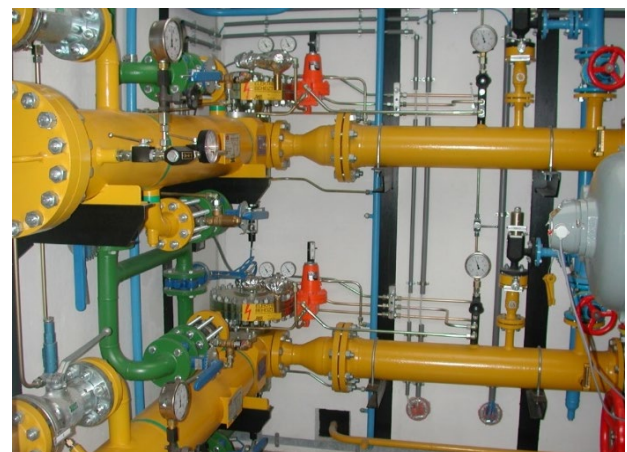
Monoblock Compact Reducing Station in concrete building with warm water heating: Flow: 2.000 nm 3 /h Pin: 20 – 70 bar Pout: 3 – 4 bar
