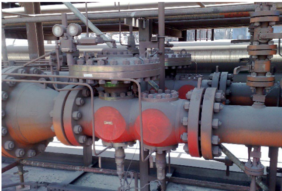
SSV / Gas Pressure Regulator under hard working conditions in cement factory
