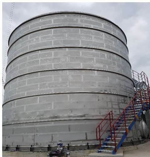
Aqueous ammonia storage tank 1.100 m 3 - site manufacturing
