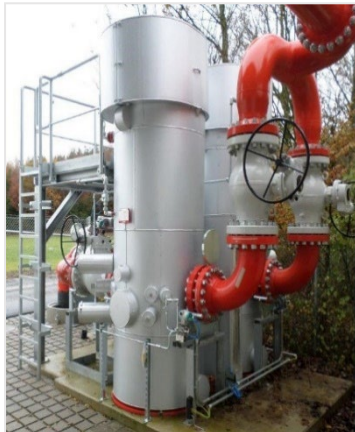
Filter Separator SNP Gas Flow 100.000 nm 3 /h; PN100
